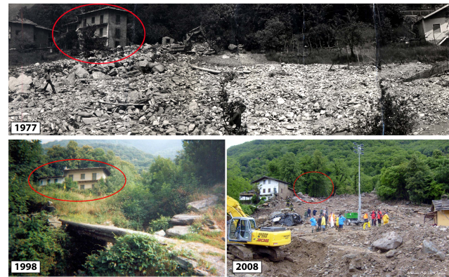
Fig. 6. Comparison of different images of the Garin alluvial fan: after the 1977 event – as the image shows, the debris flow affected a part of the fan without causing any damage to the house destroyed in 2008. In 1998 – the image shows the house destroyed in 2008 as it was until the day before the 2008 event; the image presents a very different situation compared to the following and it is particularly important because it allows us to evaluate which was the morphological context in which those who carried out an evaluation of the hazard of the area had to operate. The 2008 picture shows the post-event situation in all its drama.
