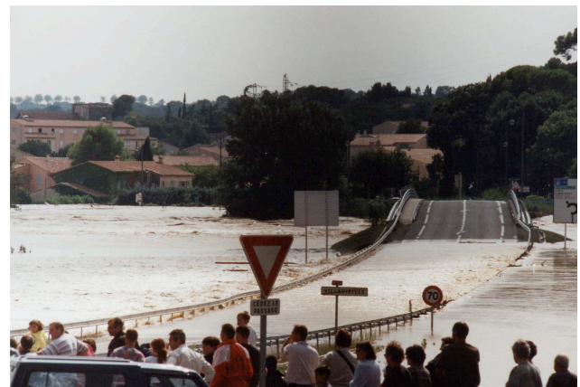
Fig. 8. Example of a submerged access road to the river crossing structure located in the flood plain (Gard 2002 flood upstream the town of Sommières).
