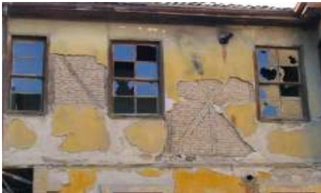
(a) Himis Structure
