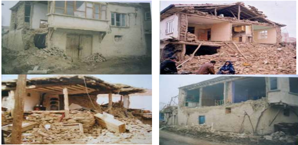
Fig. 24. Out-of-plane failure of masonry walls (Source: D. Aydin).
