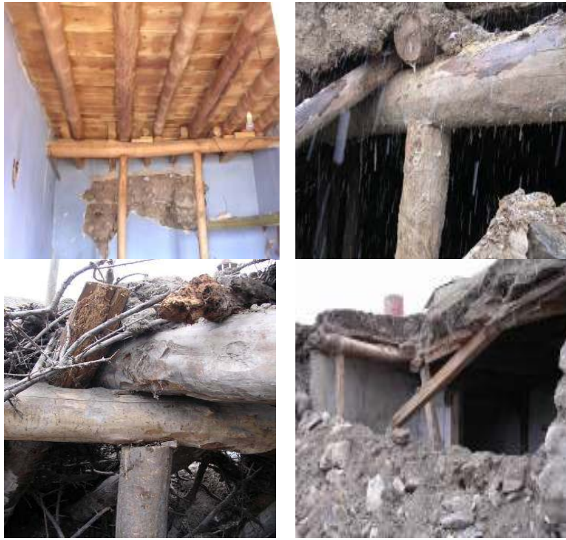
Fig. 18. Wooden frames, connection of them and failure observed in east Anatolia (Source: A. Turer).
