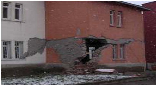
(a) Brick structure (Erzurum, 2004) (Source: A. Turer)
