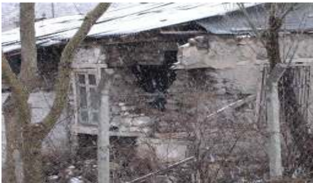
(b) Stone structure (Erzurum, 2004) (Source: A. Turer)
