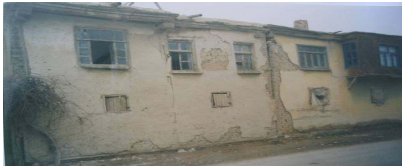
(a) Cases dwellings are constructed adjacent to each other (Source: H. H. Korkmaz, S. Z. Korkmaz, M. S. Donduren)
