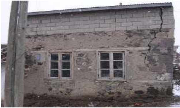
(a) Stone structure (Erzurum-2004) (Source: A. Turer)
