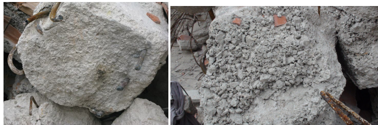
Fig. 7. Aggregate used in concrete having no particle size distribution.
