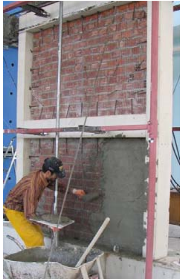
Fig. 11. Preparation of specimen SPS2.
