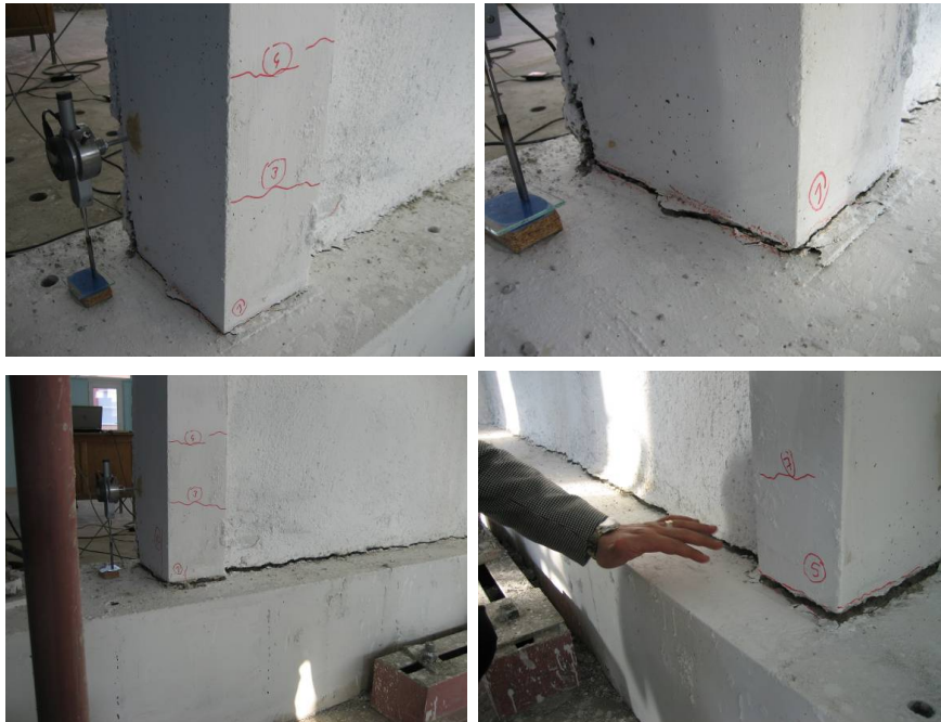
Fig. 12. Slip failures at the bottom of the columns.
