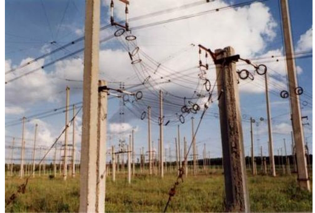
Figure 6. Elements of the heating facility antenna.
