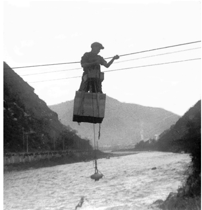
Figure 2. Stream flow measurements at gauge station Borgo a Mozzano ( 43^{\circ}59'30.73'' N; 10^{\circ}33'10.04'' E) in the River Serchio (Italy), probably taken in the 1920s or 1930s. The observer is placed in a box suspended on cable that moved along the cross section from which an old device is managed to measure the stream flow velocity (photo courtesy of Regione Toscana - Genio Civile di Bacino Toscana Nord e Servizio Idrologico Regionale).
