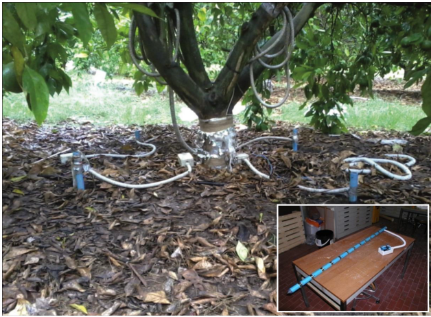
Figure 2. 3-D ERT apparatus installed around one orange tree. The system is composed of four micro-boreholes carrying 12 electrodes each (see inset) and 24 surface electrodes – see text and Fig. 3 for geometry details.
