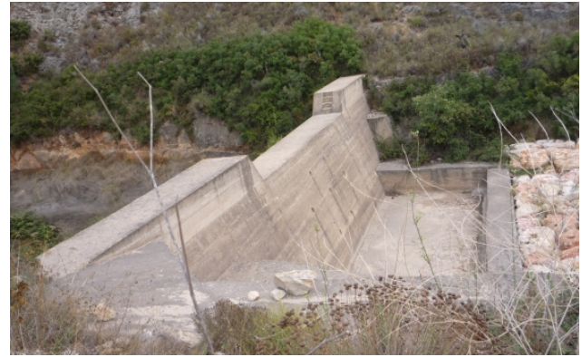
Fig. 4. The “main check dam”.
