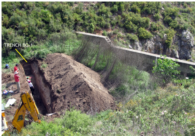
Fig. 5. The reservoir trench BG-1, closest to the “main check dam”.
