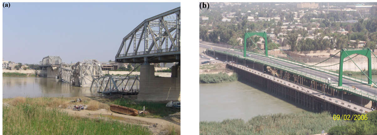
Fig. 5. (a) Destroyed parts from Al-Sarafia Bridge have fallen in the river (available at: www.wikipedia.org ). (b) Temporary bridges parallel to the suspended bridge.
