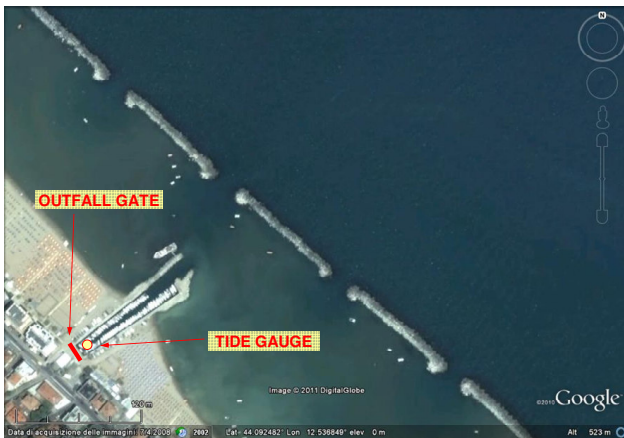
Fig. 5. Drainage network outfall and tide gauge location.
