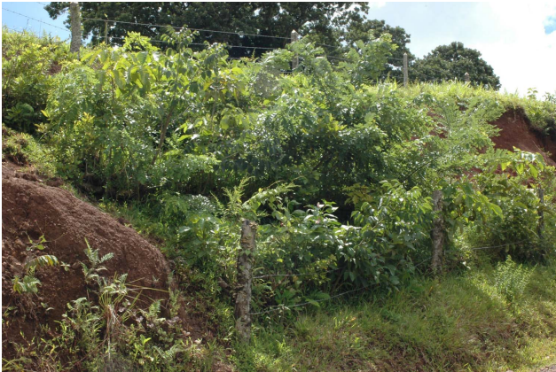
Fig. 10. The live palisade 18 months after construction.
