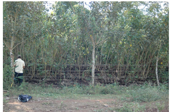
Fig. 12. The vegetated crib wall one year after the construction.
