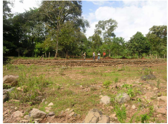
Fig. 11. The vegetated crib wall along Wanawas river just after the construction.
