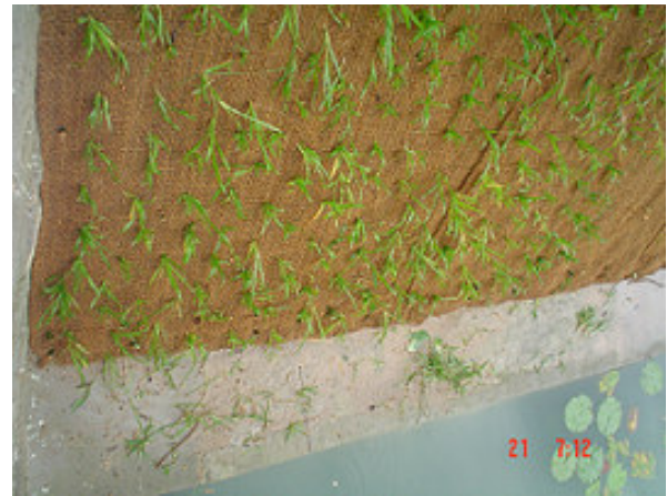
Fig. 8. CGG, third day of installation.
