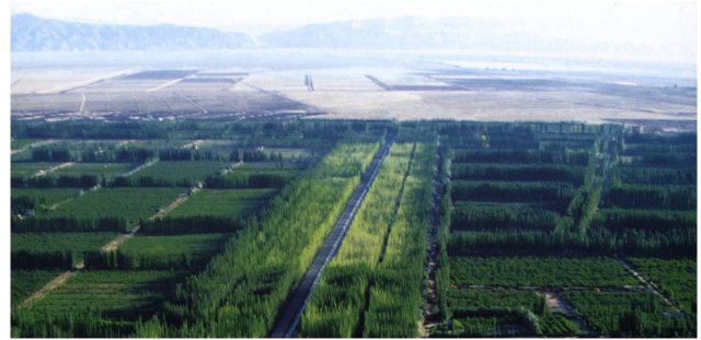
Figure 3. Aerial view of the northern edge of Kökyar I (adapted from Aksu Prefectural Greening Committee, 2006).
