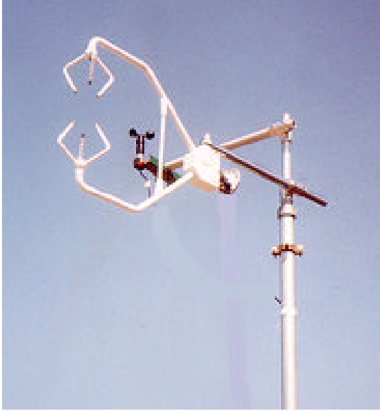
Fig. 3. Experimental mast including the sonic and the NKE cup anemometers. Heights 20 to 25 m above ground and 3.3 m above the laboratory's building roof.
