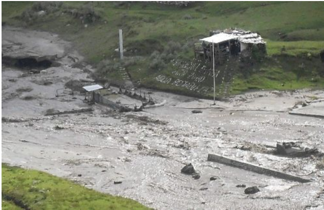
Fig. 3. Hyperconcentrated flow of 11 April 2010 at the site of the freshwater intake at Pampa Shonquil (3600 m a.s.l.). The structures have been completely inundated and partially damaged (mainly through erosion and deposition of material). Photo by Arq. Luis Meza, Carhuaz.
