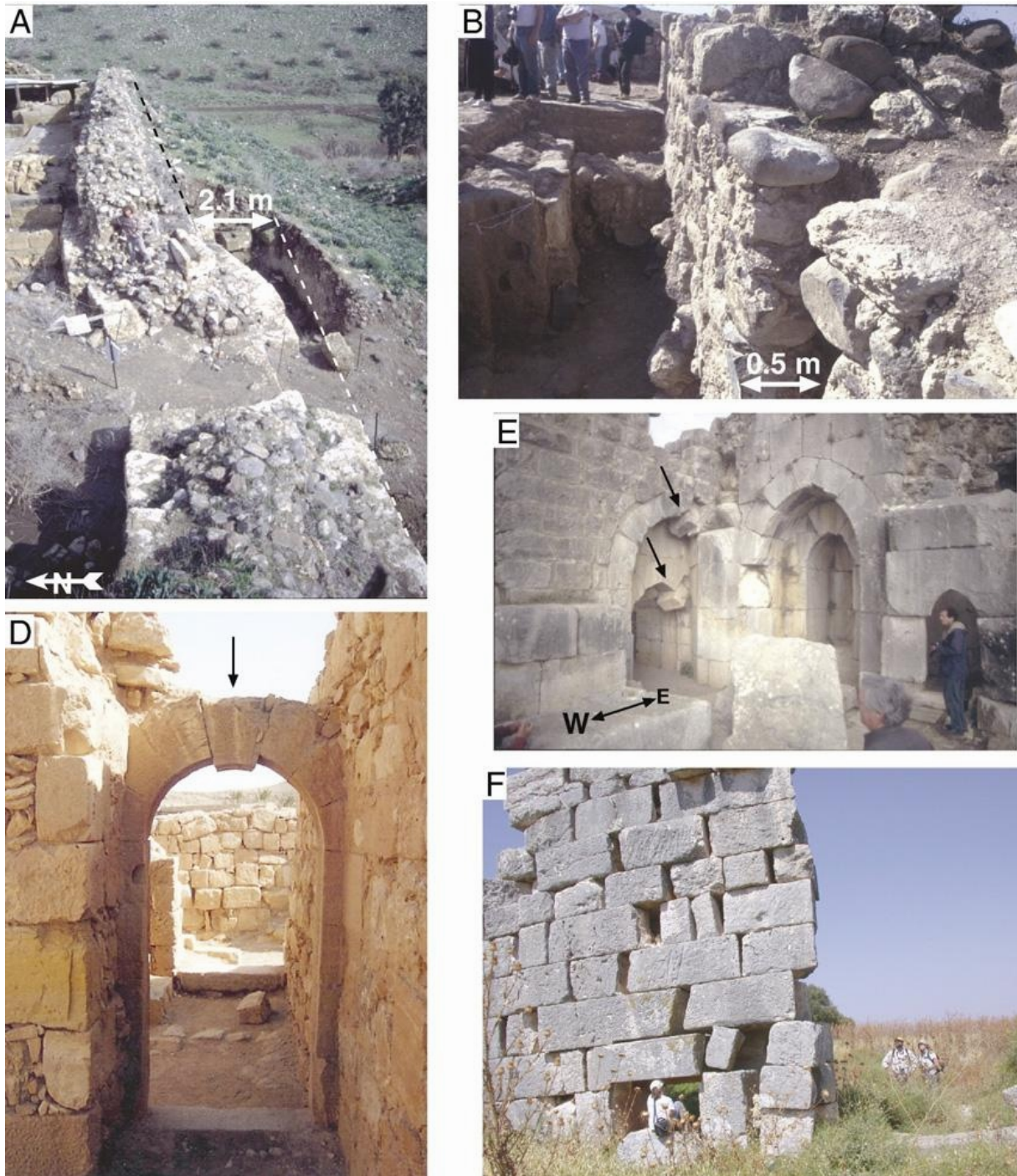
Fig. 4. (A) An offset wall of the Crusader fortress of Vadum Iacob. Dashed line shows original geometry. The 2.1-m-offset is the sum of 1.6 m and 0.5 m displacement caused by the earthquakes of 20 May 1202 and 30 October 1759, respectively. (B). An offset wall of the Ottoman Mosque that is built on top of the Crusader fortress of Vadum Iacob. The associated earthquake occurred on October 30, 1759 (C). A water trough in Um el Kanatir left-laterally offset about 1 m on the margin of a landslide triggered by the earthquake of 18 January 749 (D). A keystone slid down in an arch enclosed symmetrically by a wall (photographed in Mampsis) (E). Blocks on the sides of arches on the left slid down in the earthquake of 1759 in Kal'at Nimrod. Throughout the site, arches in walls that trend E-W are deformed whereas similar arches in N-S trending walls have remained intact (F). Horizontal shift of large ashlars in the Hellenistic temple of Kadesh (site occurred in the 749 earthquake). All these sites occur in Northern Israel (after Marko, 2008).
