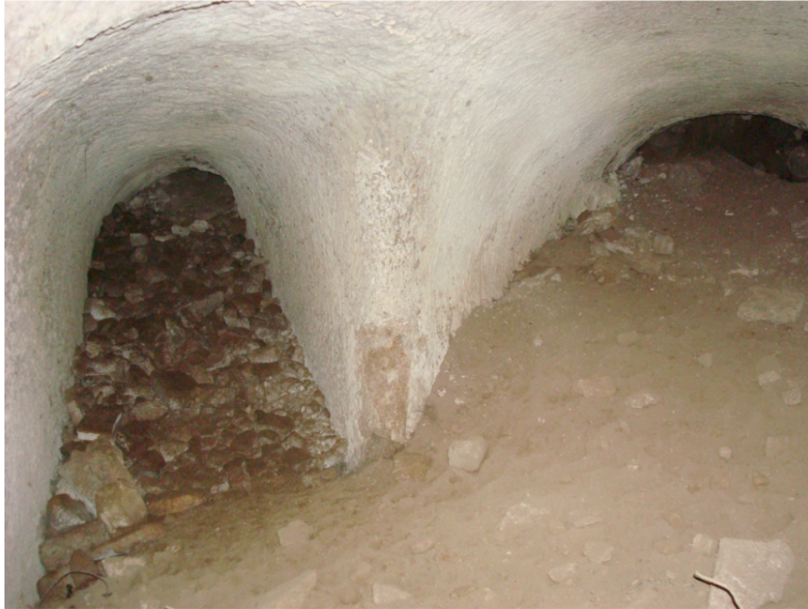
Fig. 6. The last accessible part of tunnel C, where it splits in two different galleries (photo M. De Franceschini).
