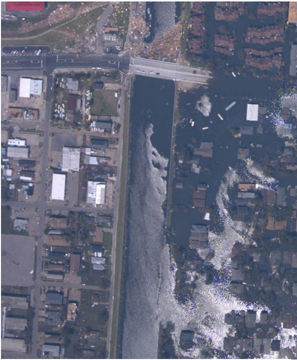
Fig. 5. Breach in 17th St. Canal in New Orleans, LA, 31 August 2005. Credit: NOAA.
