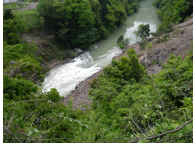
Fig. 6. Debris deposits in the river course (14 May 2006).
