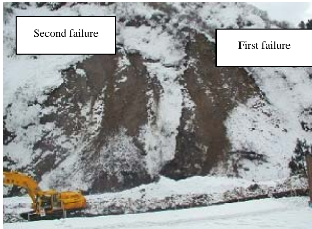
Fig. 1. Slope failure on left bank of the Sanashi river.
