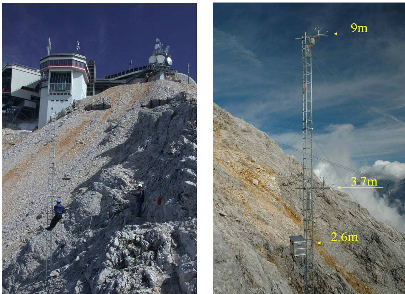
Fig. 3. Photographs showing the two masts, one on the northern side (left panel) and the other one on the southern side (right panel) of the ridge. The view is from the southwest looking upwards toward the summit of Mt. Zugspitze. Measurements at each mast are taken at two heights, namely 3.7 and 9 m above ground.
