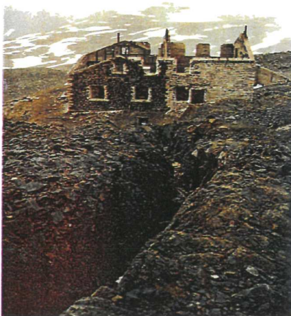
Path from the living house to the Observatory blast down in the rock in order to prevent the observer not to blow away
