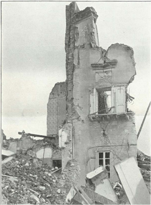
FIG. 8. Ruin of French Consulate. Walls fairly thick and well built but floors weak and house too high for this type of construction.
