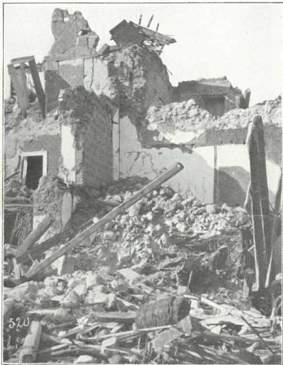
FIG. 6. Showing rubble construction.
