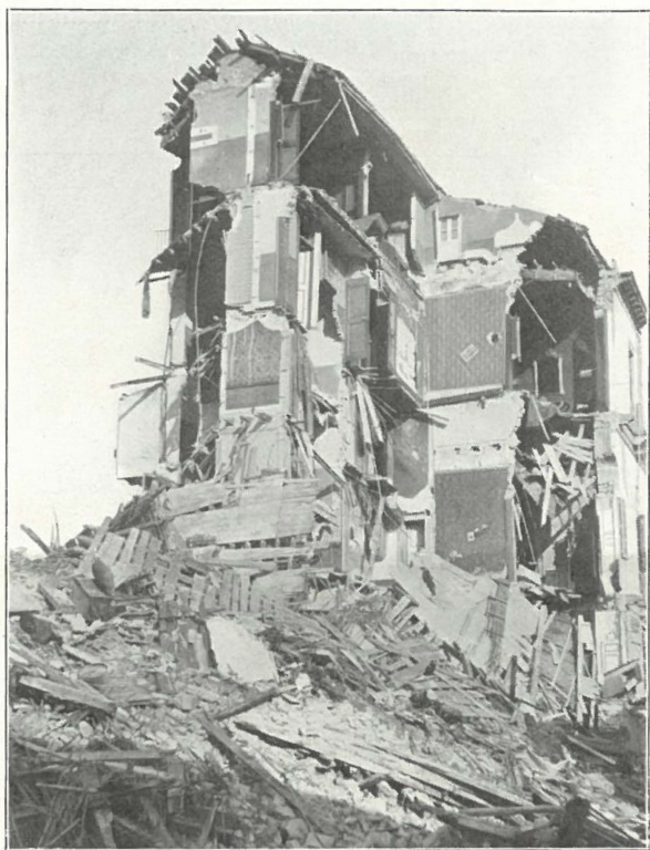
FIG. 13. Wreck of a tall, poorly constructed building.
