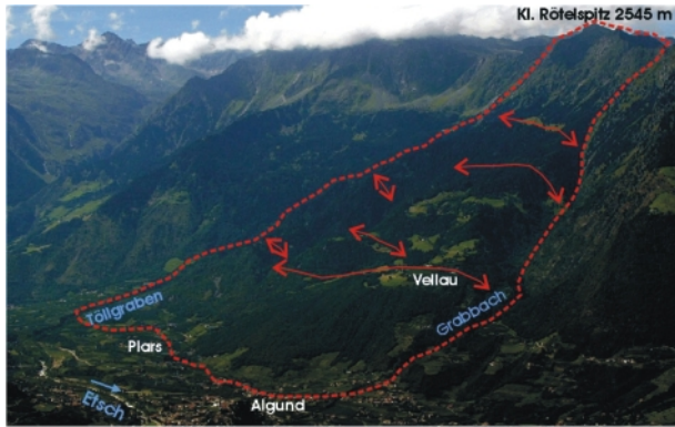
FIGURE 3: View of mass movement “Talzuschub Algund”, with red dashed line indicating rock mass affected by the creeping movements and solid red lines indicating major scarps/trenches related to the sagging/complex rock flow (see also Figure 4).
