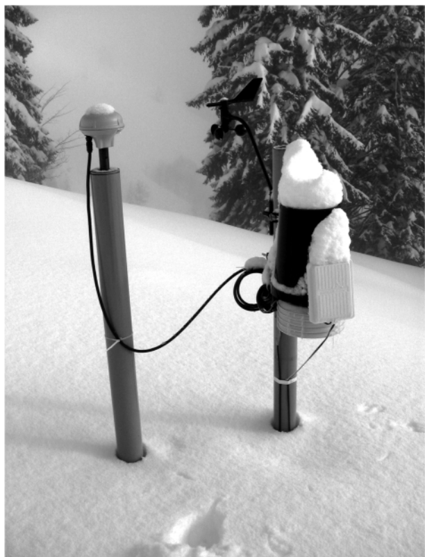
FIGURE 12: Winter impressions at Aggenalm test site. Main sensor node with GNSS sensor (Novatel Smart V1G-Antenna) and weather station.
