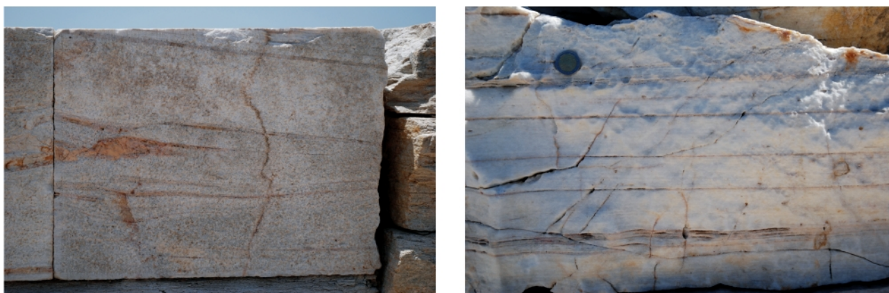
FIGURE 7: Comparison between building stones with outcrop lithologies on Despotiko. a) Two building stones from Building A consisting of marble 1 (centre and left part) from the east façade of room A1. Note the carefully dressed surfaces, the white, slightly greyish colour and especially the characteristic rose-coloured layers of fine grained dolomite marble. The building stones below and to the right comprise white mylonitic gneiss. b) Outcrop photograph of marble from Cape Koutsouros (for location see Figure 3), comprising white, medium grained calcite marble with well developed foliation and characteristic rose coloured, thin dolomite marble layers. Note the close similarity with marble 1 from Building A (for colours see the online version of this paper).
