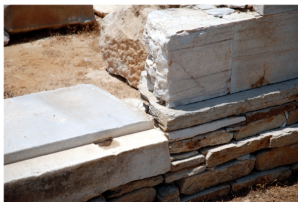
FIGURE 6: East wall of room A2. The large threshold on the left comprises the massive, coarse grained, slightly greyish marble 2. Marble 1 of the well dressed building stones of the east façade is easily distinguished by its well developed foliation and thin, rose-coloured dolomite layers. Foundation stones are made of white, strongly foliated, mylonitic gneiss. Several orange-brown coloured fractures indicate that the stones have been separated in the quarry along the fractures and these fracture surfaces have hardly been modified later (for colours see the online version of this paper).
