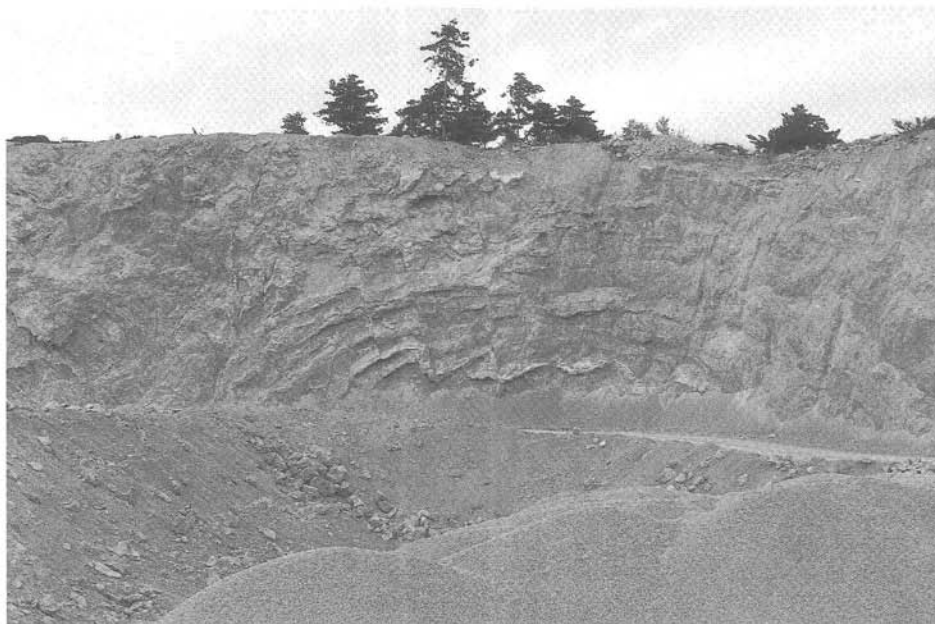
Fig. 164: Fold with a SSW dipping axis within the Hauptdolomit. The faults are marked by mylonitic, cemented zones. Quarry Baukontor.
