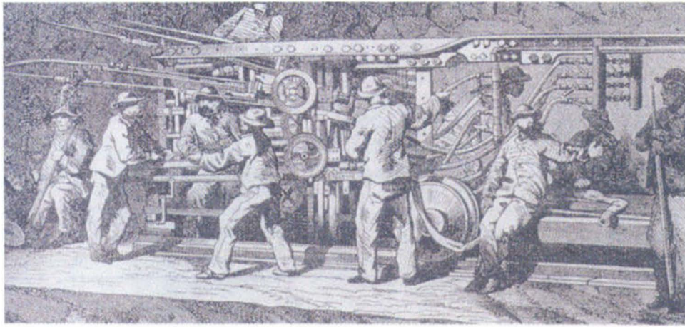
Fig. 3. The Sommeiller drilling machine designed for the Mont Cenis tunnel.
