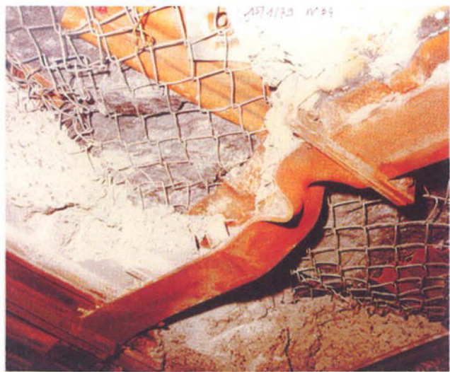
Fig. 17. The Frejus Tunnel : The failure of heavy support with steel arches and concrete.
