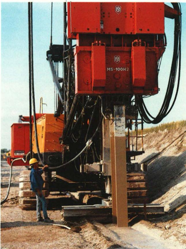
Abb. 7: Schmalwandherstellung Fig. 7: Thin diaphragm wall construction (vibrated beam slurry walls)
