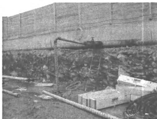
Abb. 10: Jet-grouting Wand, Anker, Brunnen
