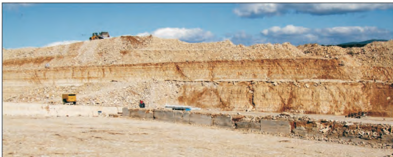
Fig. 26: A modern technology in the Benkovacki Kamen quarry enables making long vertical walls and exposing large bed surfaces.
