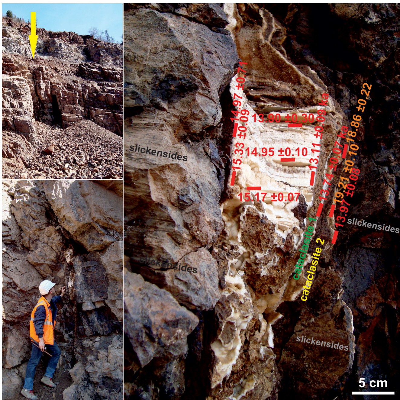
Text-Fig. 14. Brittle fault (damage) zone hosting two major vertical fractures in the southern part of Erzberg both entirely sealed with erzbergite carbonate (level Schuchart, ~1,110 m a.s.l.). The northern (left) fracture features slickensides and two generations of cataclastic rocks. Multiple and precise ^{238}\text{U} - ^{234}\text{U} - ^{230}\text{Th} age data of the aragonite precipitates support young ages ( < 20 kyr BP) and rapid deposition of the \text{CaCO}_3 filling the fracture and cementing the cataclasites. The latter are mostly in original position and can be traced for several meters in the downwards narrowing fracture. The petrographic and structural characteristics of this place in combination with the radiometric dating results raise questions on a geologically young age of the fractures/faults and cataclastic rocks, as well as the possible reactivation of directed rock movements.
