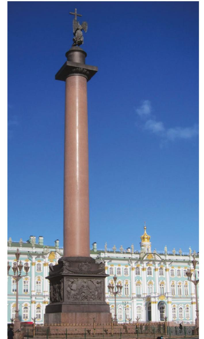
The monolith and the pedestal of Alexander Column (1829–1834) are made of Virolahti pyterlite. Photo: Paavo Härmä.
