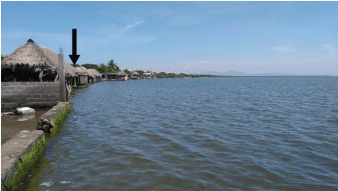
Figure 1. Tectonic subsidence, IX ESI-07 . Area of restaurants flooded by sea water. Juchitán, Oaxaca.
