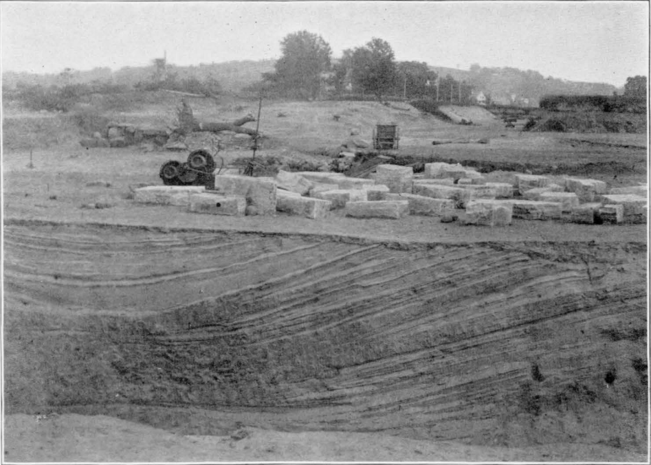
FIGURE 1.—GENERAL VIEW OF CUT AT NAVY YARD, LOOKING SOUTH
