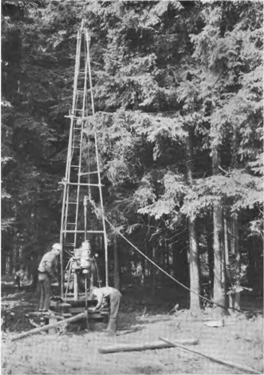
110. Core drilling 1967/2, summer 1967
