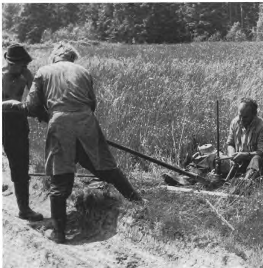
11. Top hardrock checked by "needle" tests, summer 1967
