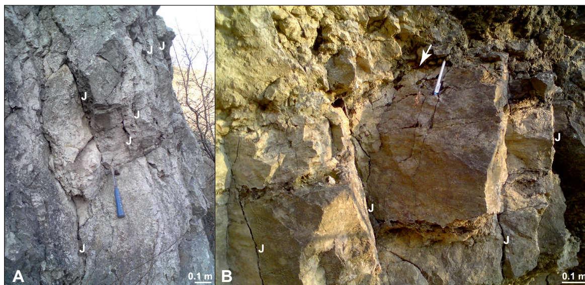
Fig. 10. Outcrop views of the Hollingstein Limestone from the abandoned quarry at the Steinberg. A — North-western wall of quarry. B — North-eastern wall of quarry, transition (arrow points to boundary) from Hollingstein Limestone (lower part) to nodular limestone blocks and fragments of the Blocky Layers. Note the dilated joints (J) in both figures pointing to extensional strain during transport of the olistolith.
