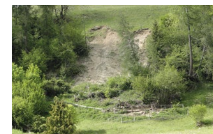
Hangrutschung in Siedlungsnähe. Landslide near a settlement.
