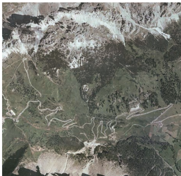
Fig. 5: Aerial view of the Passo Gardena landslide.
