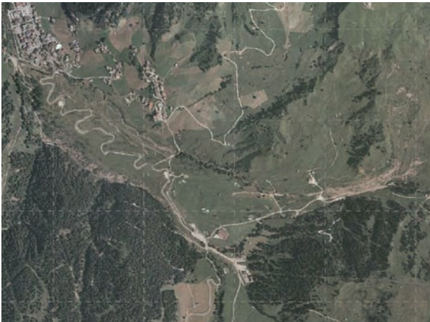
Fig. 6: Aerial view of the Corvara landslide.
