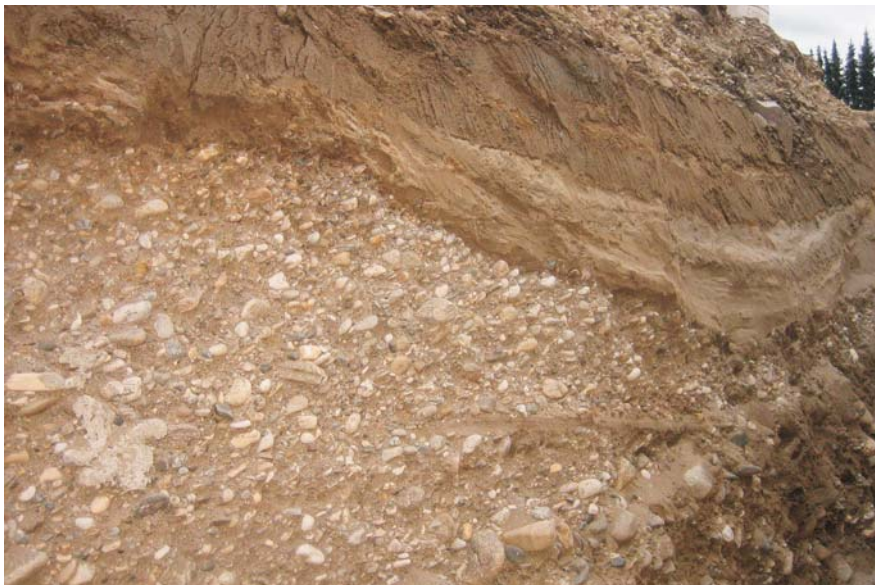
Baugrube in der Stadt Graz. Building pit in the area of Graz.
