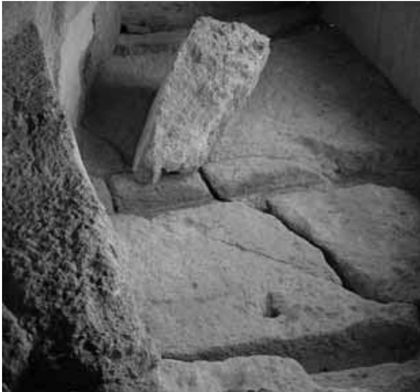
Figure 21 - Internal view of the Church, with the fractures and blocks outcrop.
