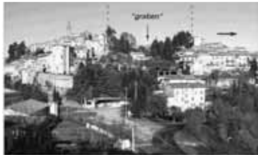
Figure 23 - Graben structure (the horizontal arrow indicates the moving part of the village)
