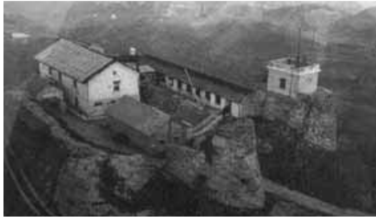
Figure 54 - A photograph likely taken after the 1930 earthquake, where it is possible to observe the same fracture observed in 1980 cutting the stairs of the observatory building.
