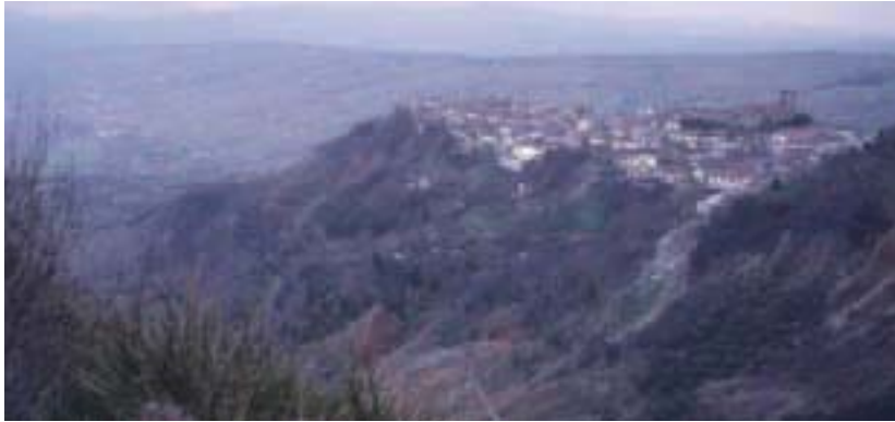
Figure 49 - The high escarpment which divides the old town from the modern one (out of the picture, on the right side). Secondary escarpments are visible within the built-up area. All of them can be interpreted as landslide scarps.
