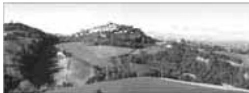
Figure 22 - Frontal view of the landslide area
