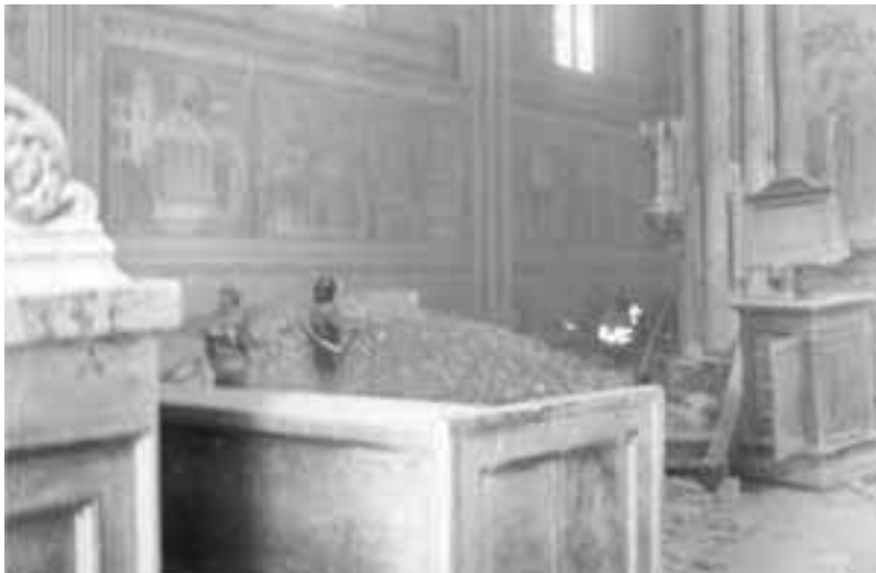
Figure 4 - Firemen working among the ruins after the fall of the ceiling upon the major altar.
