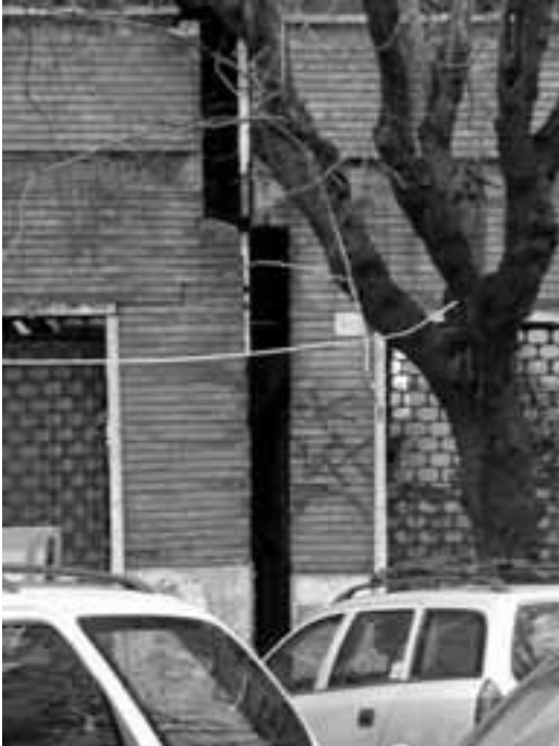
Figure 2.24 - The S. Paul area: detachment of two originally adjoining buildings because of differential settling.
