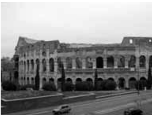
Figure 3.4 - Southern side of the Colosseum, where most of the seismically-induced damages have occurred. The first two rings are missing and the third one, which collapsed after the 1703 earthquake, was reconstructed only in 1845.
