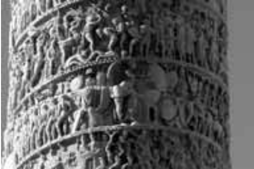
Figure 3.7 - Mismatch of drums (detail of Figure 3.6).
