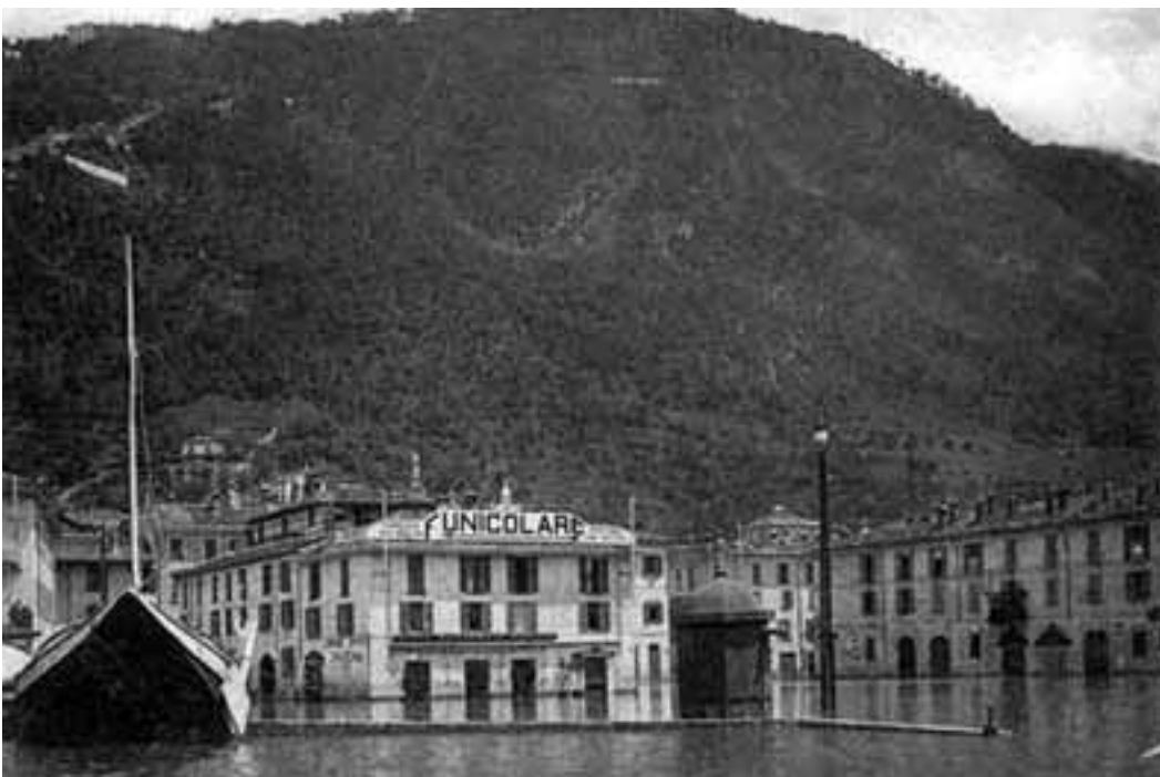
Figure 1.9 - The Brunate hill and the Como funicular station during the 1910 lake flood.
