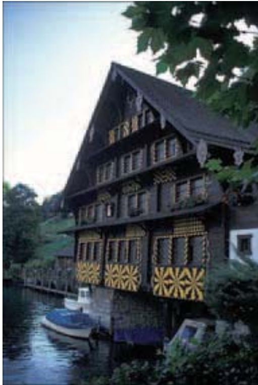
Figure 3.8 - Gasthaus Treib, which was flooded by the 1687 tsunami, up to the 2nd floor.
