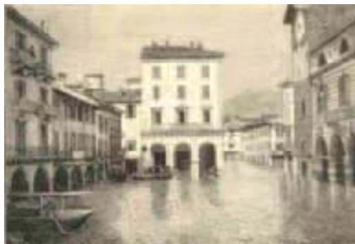
Figure 1.11 - 1888 lake flood in Piazza Duomo.
