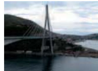
Figure 6.7 - The bridge over the Rijeka Dubrovačka.
