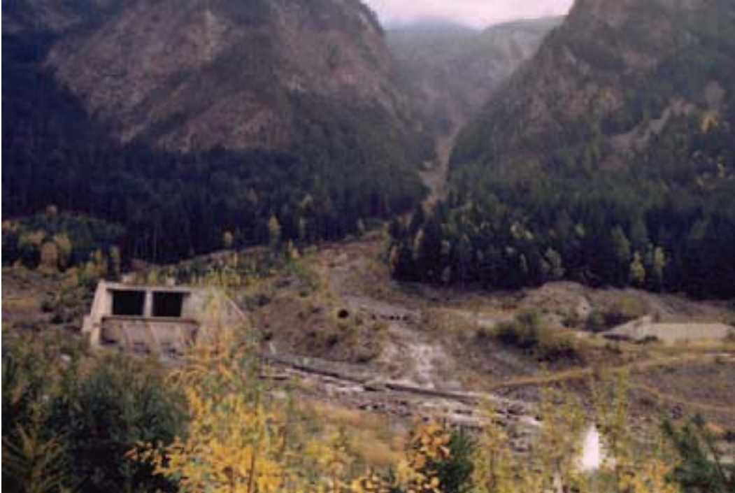
Figure 28 - The exit of the bypass tunnels, situated downstream the Valpola landslide, near locality "Le Prese".
