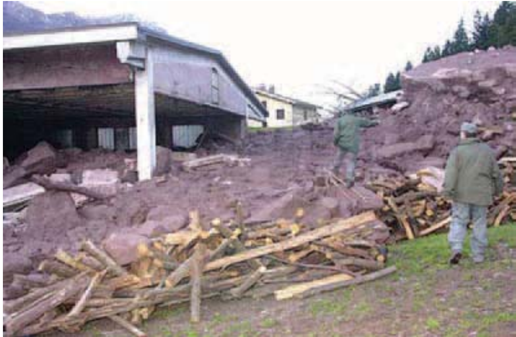
Figure 19 - Damages to buildings and factories in Bindo area
