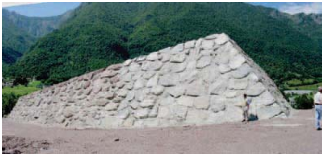
Figure 16 - Diversion cone placed near the top of the alluvial fan in the Rossiga Torrent, built to protect the hamlet of Galera.
