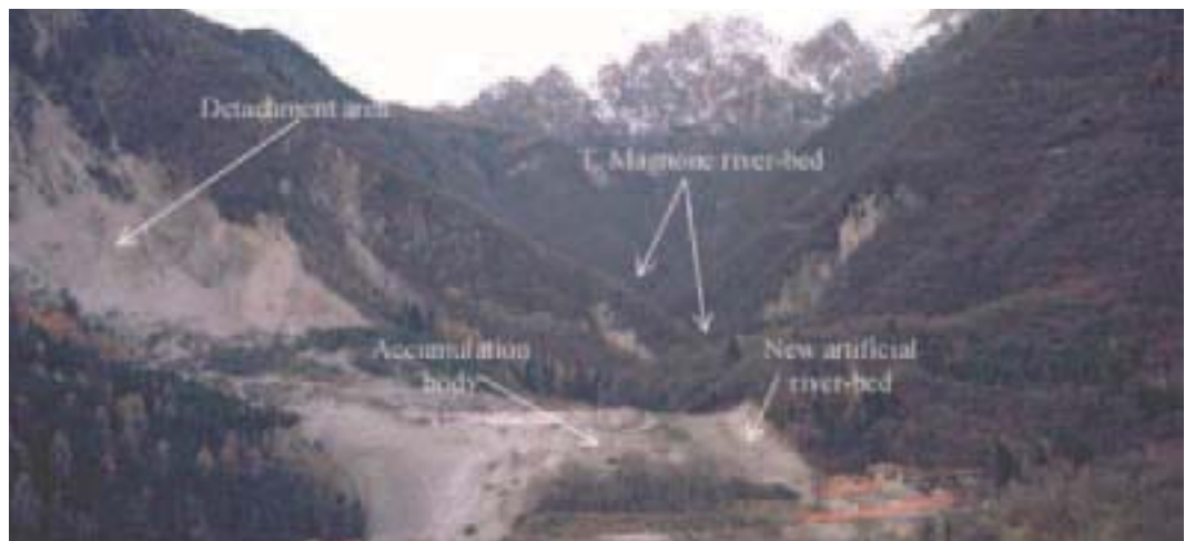
Figure 66 - Tenno landslide panoramic view. The houses damaged by the landslide can be seen on the right of the accumulation body while the main scarp is visible on the upper left. The length of the landslide is about 400 m and its width is more than 200 m. The estimated volume of the displaced material is about 4 M m 3
