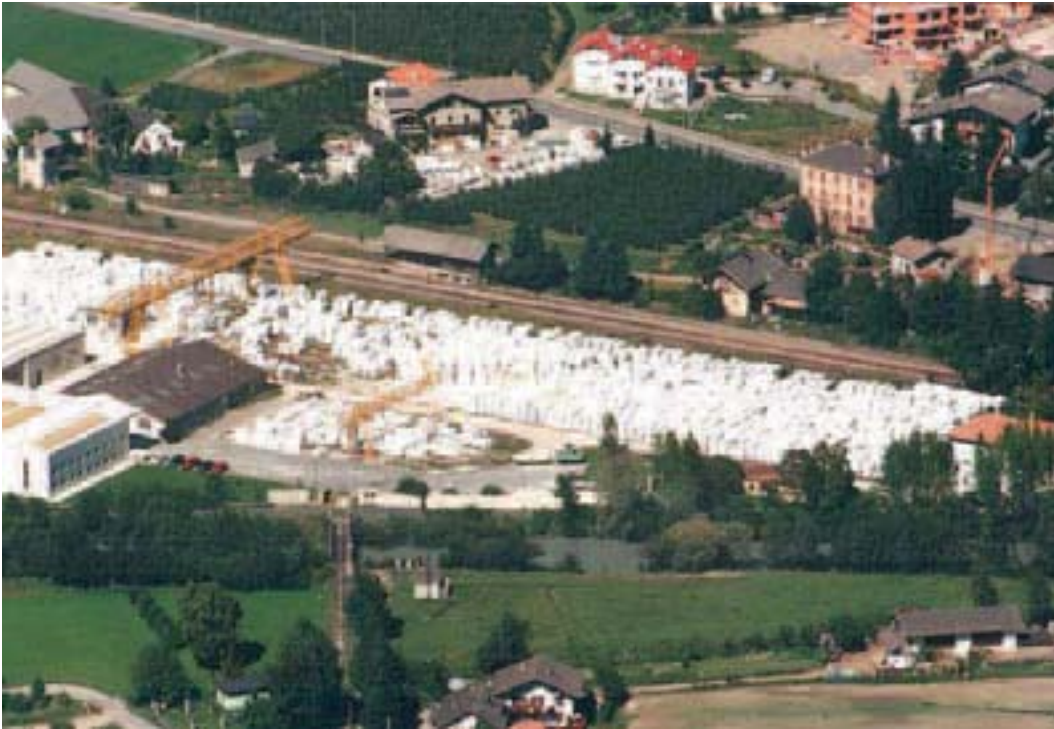
Figure 38 - The Lasa marble factory viewed from the upper station of the funicular that carries marble blocks from the mine to the working place.
