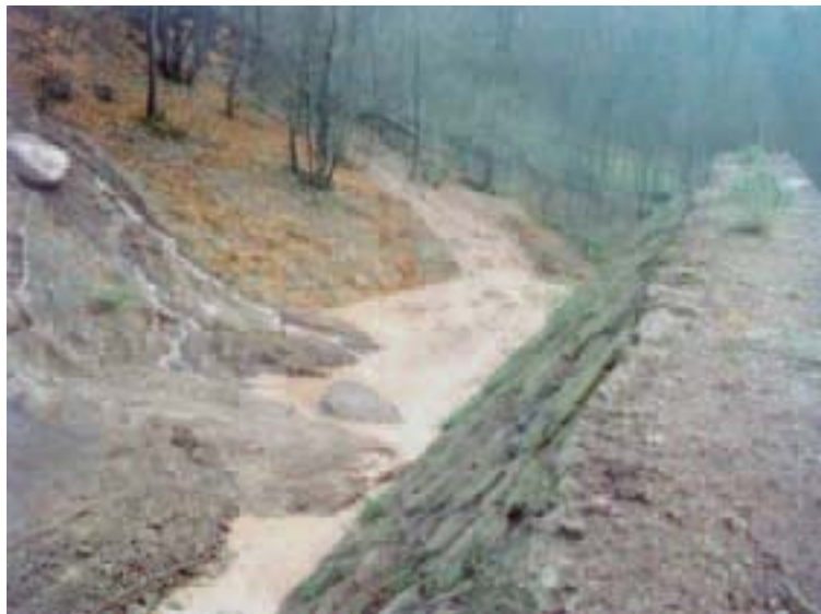
Figure 13 - The water arriving at the bottom of the slope was becoming more and more turbid presaging an imminent landslide
