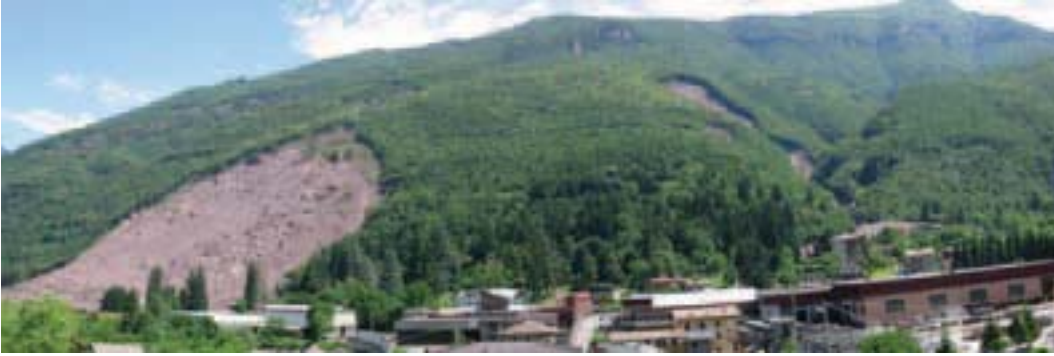
Figure 17 - Panoramic view of the landslide area above Cortenova village: on the left, the collapse which struck the hamlet of Bindo, and on the right, a glimpse of the area where the debris flows originated
