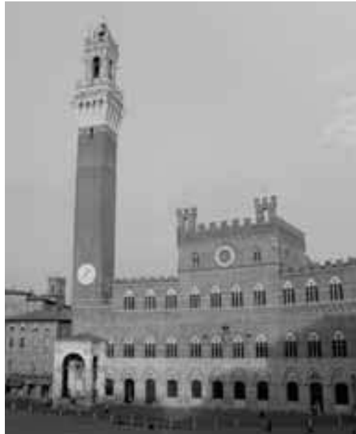
Figure 7 - Palazzo Pubblico and Torre del Mangia.. Note stratification of different bricks used during construction.
