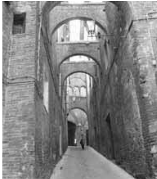
Figure 9 - Arches in Via della Galluzza built to protect old building against earthquakes
