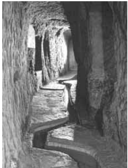
Figure 6 - Meandering path of a gorello to locally slow down and deepen water flow to ensure constant water distribution to intersecting gorelli of utenze (clients).
