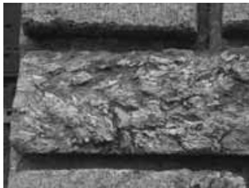
*Figure 12 - Facies 3 selenitic gypsum in a block of the Garisenda tower of Bologna.*
