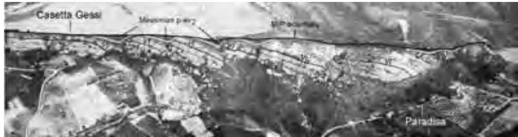
Figure 28 - Air photo of the Vena del Gesso in the western side of the Santerno Valley (M. Astorri). Normal faults and very small reverse faults offset the evaporite cycles, and are sealed by post-evaporite Messinian deposits, which mark a spectacular angular unconformity. The rotational offset of faulted blocks suggests gravity-driven normal faulting, gliding and thrusting on a shallow detachment level within the euxinic shales. Transport was to the S-SW.
