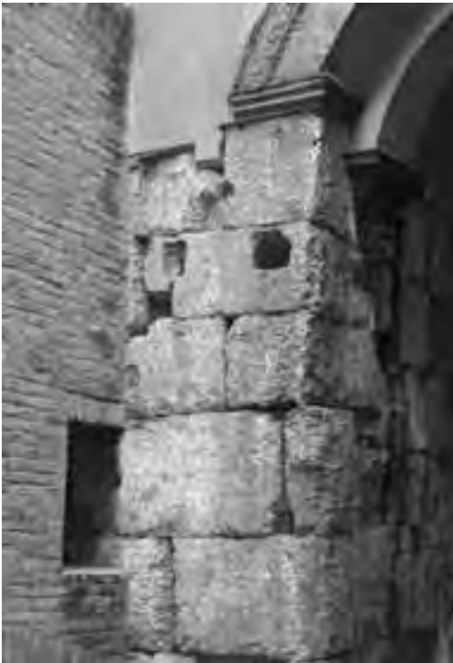
Figure 1 - Remnants of the IV-VIII century AD selenite walls, preserved and recycled in the Ghisilardi Fava Palace at Bologna .
